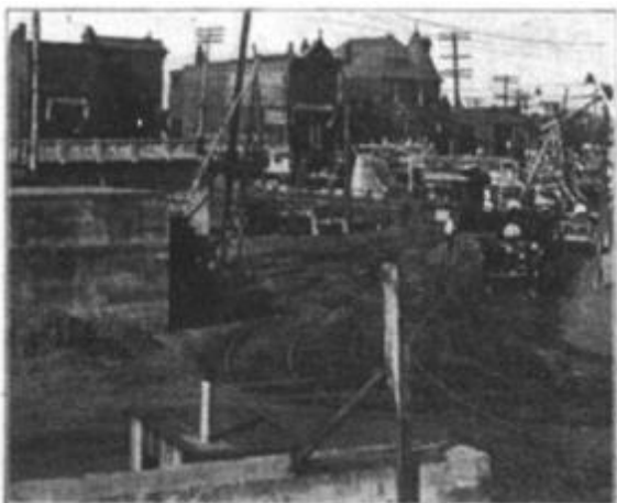
Construction View Showing Conditions Before Grades Were Separated
