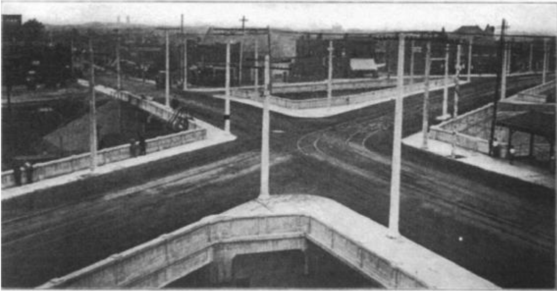
Overhead View of the Viaduct Looking North
