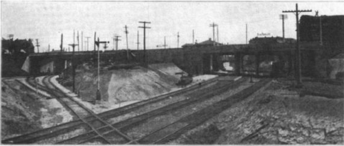
West Elevation. Frisco Tracks on the Right Crossing Missouri Pacific Oak Hill Branch in the Foreground
